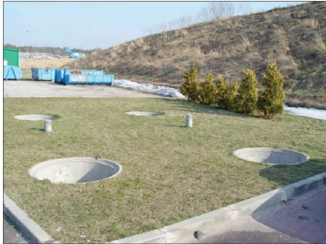
Figure 3.3 Tanks for leachate from landfill, composting plate for green waste, and slope of old landfill.
