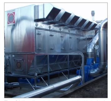
Figure 2.1 Sleeve filters air-cleaning system AAGAARD. Produced in Denmark, in 2001.
