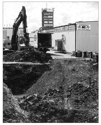
**Figure 2.2 Remediation of soil.** Old filling stations are sites where the soil is routinely monitored for chemicals before new uses. Here the soil under a previous gas station is being removed for a new residential house. (Photo: Lars Rydén)
