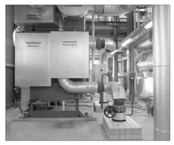
**Figure 6.8 Using heat pumps.** This large industrial heat pump is taking its heat from the flue gases from waste combustion at Vattenfall, Uppsala Energy. In the process the gas condenses and the heat extracted is transferred to the district heating system. In other large-scale applications heat is extracted from sewage water or surface water. The chilled water may be used for district cooling. Most heat pumps are smaller and used for individual homes. (Photo: Kjell-Arne Larsson)
