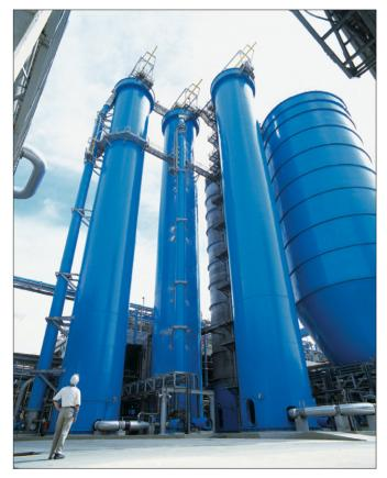
Figure 2.6 Bleaching towers in a Kraft Mill System. The sulphate process, also called the Kraft pulp process, is a recovery process, where the chemicals used in the cooking of the pulp are, generally, recycled. In addition so-called black liquor produced in the process may be incinerated and as such provide the industry with all energy needed. (Photo:  $\bigcirc$  Andritz AG)
