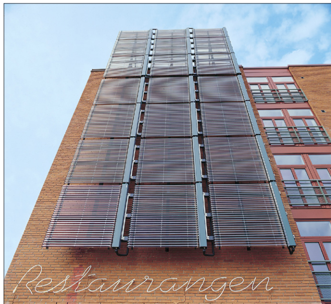
Figure 4.3 A solar collector balcony (Example 3). This balustrade is used both as a solar panel and as a balcony balustrade. The Vitosol 200 model is found in the City of tomorrow (Bo01 exhibit in 2001) in Malmö. Photo: Viessmann Werke GmbH & Co KG.
