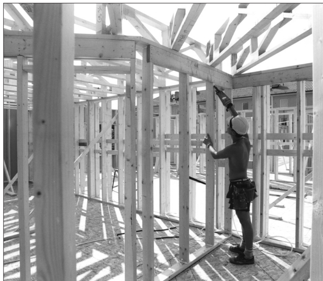
Figure 3.1 Multi-storey wooden houses. One of the many advantages of multi-storey wooden houses, here being built outside the Swedish city of Norrköping, is many times lower consumption of the natural resources, less handling of heavy material, easy transport etc. Photo: Holger Staffansson, Skanska.
