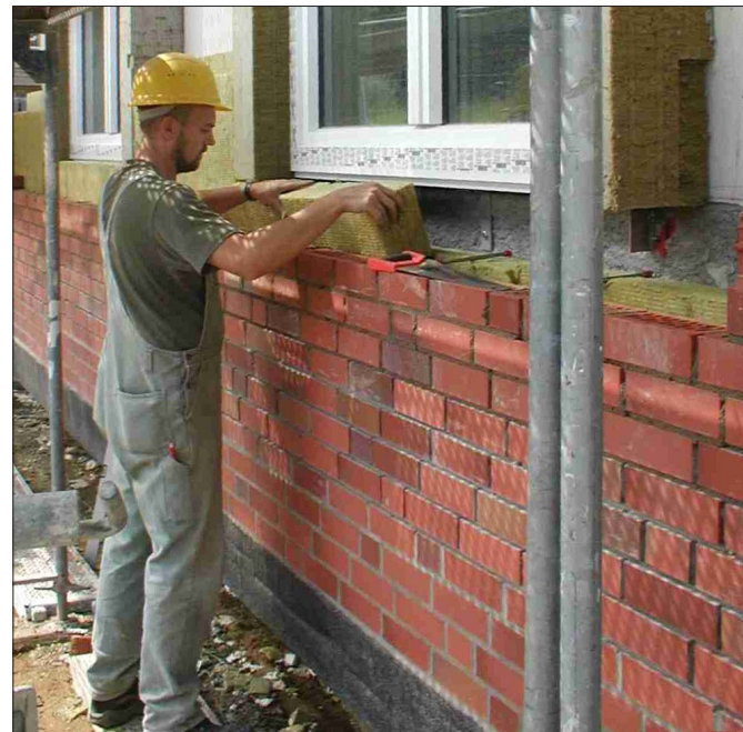
Figure 3.3 Building of a passive energy house. The house is insulated to achieve a U-value that does not exceed 0.15 \text{ W/m}^2\text{K} ( 0.026 \text{ Btu/h/ft}^2/^{\circ}\text{F} ) which typically corresponds to 20-40 cm of insulation.
